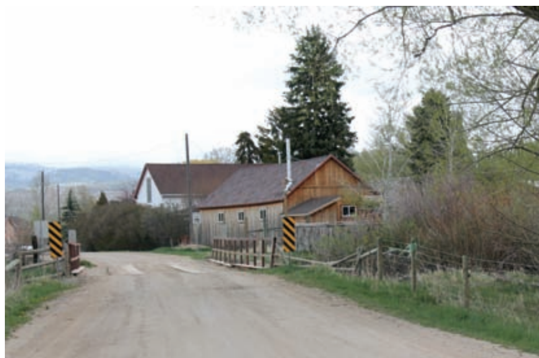
CAITLIN AVEY/THE MADISONIAN Once Blaine Spring Creek and Varney bridges are replaced, the county has prioritized Laurin Bridge as next on the list.
