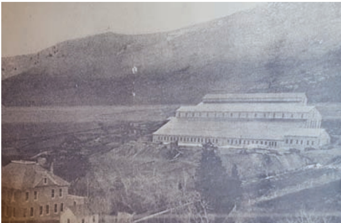
PHOTO COURTESY ANNE PHILLIPS REYNOLDS The old stamp processing mill was built during the mining boom when the grade of ore was determined to be high. The ore body turned out to be of low grade and the mill never actually ran.
