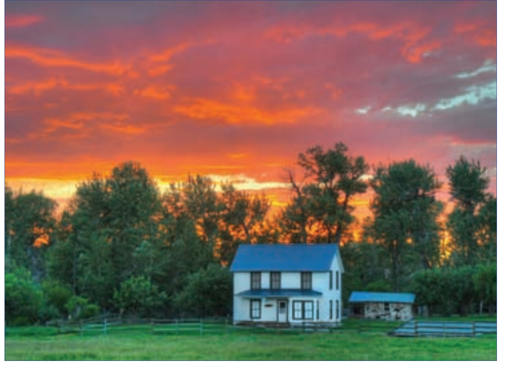
The Fenton House during the summer of 2012.
